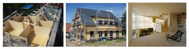
Figure 2. Examples of buildings using CLT panels (Mestek, Werther & Winter, 2010)
