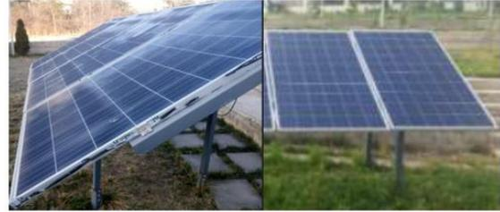
**Figure 2.** PV panels placed with an optimum annual angle of 34°.
